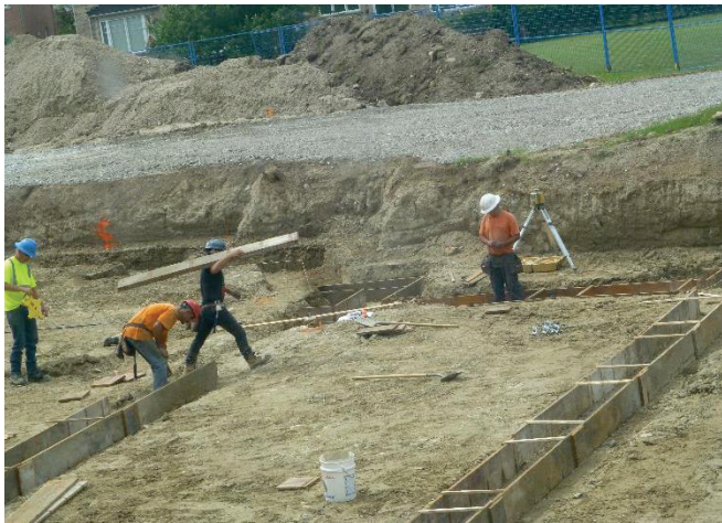
Building the forms for the footings & foundation
