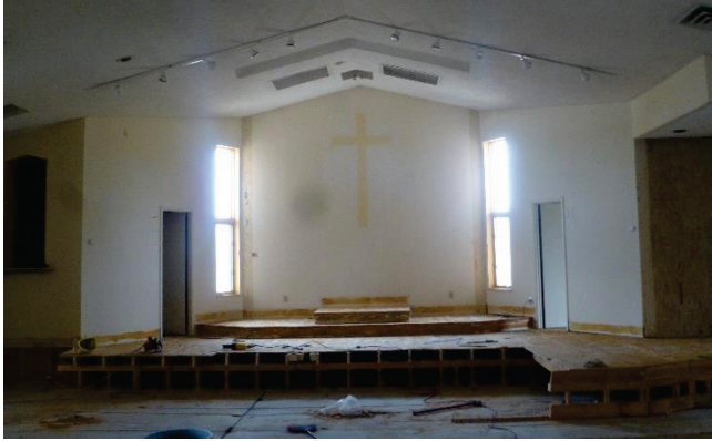
Demolition of the sanctuary floor
